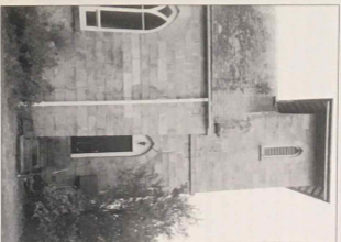
THIS VIEW OF THE TOWER SHOWS THE CRACK THAT HAS DEVELOPED AND THE SLIGHT LEAN IT NOW HAS.
